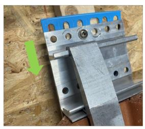
The roof hook must be fastened to the rafter with two screws. The shim plate is flush with the base profile of the roof hook.
