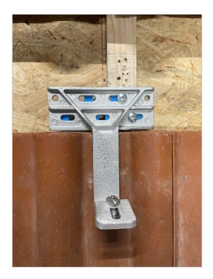
The roof hook must be fastened to the rafter with two screws.
