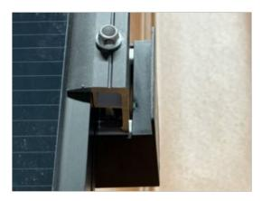
The picture on the left shows the fully assembled end cap for the C-rail.
