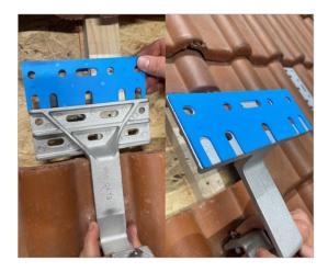
The shim for roof hooks must be positioned precisely under the base profile of the roof hook.
