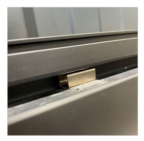
The contact latch must be firmly seated in the rail.
