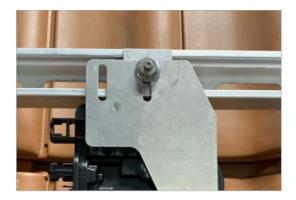
The rail nut is screwed into the C-rail
